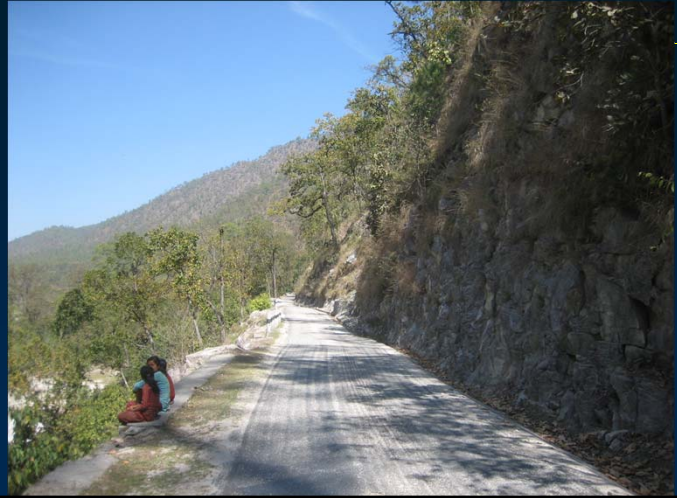
Dam Site- Left Bank
