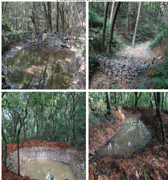
Figure 3: Different types of recharge ponds constructed in Thuloban, Dhulikhel
