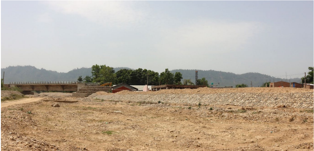
Photo 17: Ongoing bridge construction in Mahadewa River with the nearby houses below the riverbed
