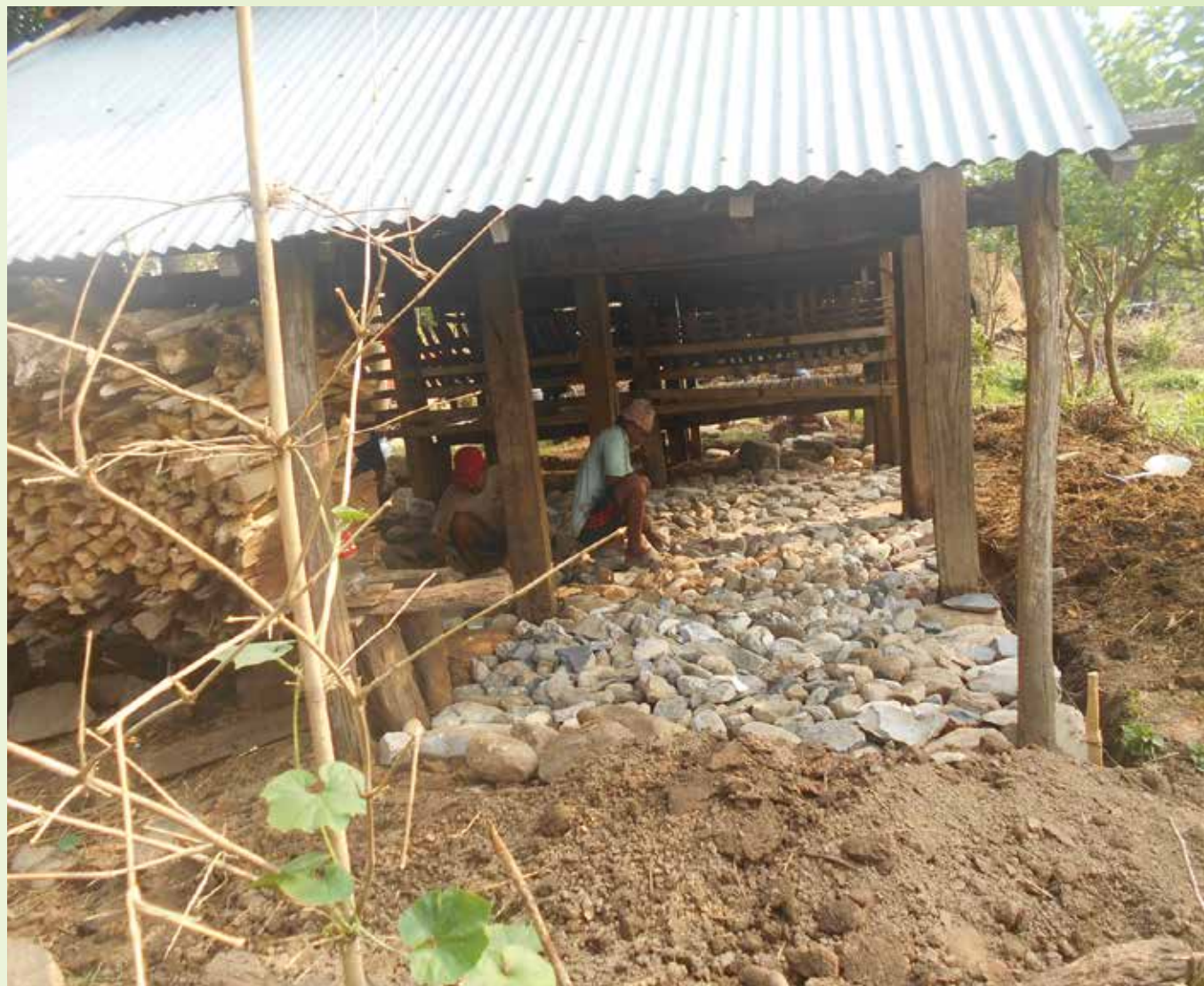
Cattle shed under construction
