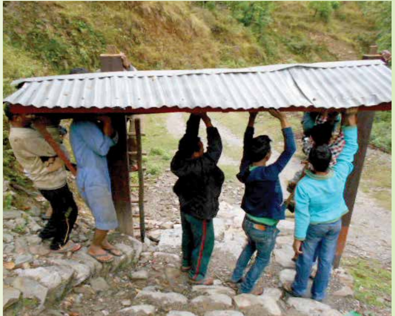
Locals repair Khasur Gate
